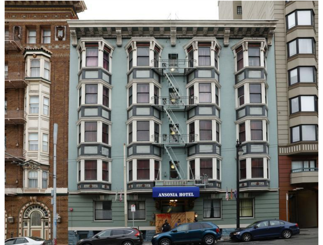
711 Post Shelter Photo Credit: SF Examiner
